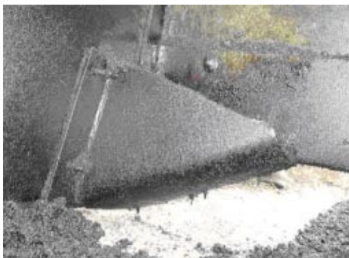
A special edging device on resurfacing equipment creates the “Safety Edge”
