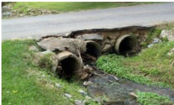
**A headwall structure may have prevented the soil erosion and subsequent loss of pavement structure pictured at this three-barrel precast concrete culvert.**
