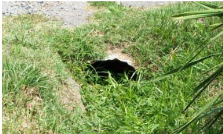
**This corrugated metal culvert displays a significant loss of capacity due to excessive sedimentation both in the culvert itself and in the ditch leading to the culvert inlet.**
