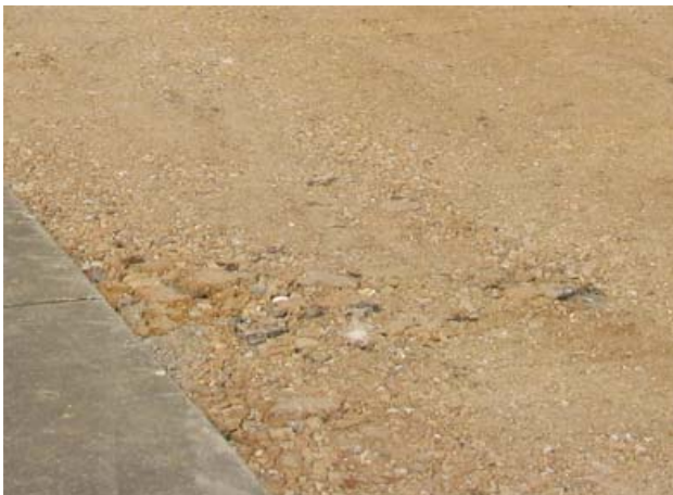
Figure 3 – Cement Over Graded Material
