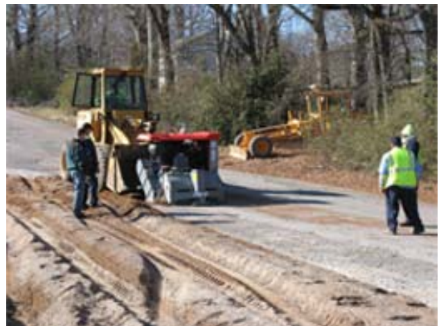
Figure 2 – Pulverization with Asphalt Zipper
