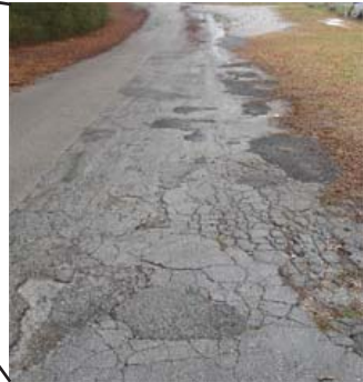
Figures 1a, 1b, and 1c – Pavement Areas with Severe Distress & Poor Drainage
