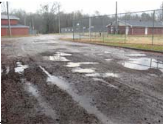
Figures 1a, 1b, and 1c – Pavement Areas with Severe Distress & Poor Drainage
