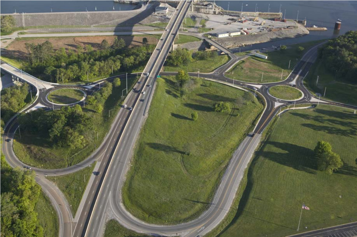
Two new multilane roundabouts accommodate the intersection of Lake Resort Road, North Access Road, and Tennessee State Route 153 in Chattanooga. This design alleviates congestion while accommodating for the replacement of the lock at Chickamauga Dam, shown in the background.
