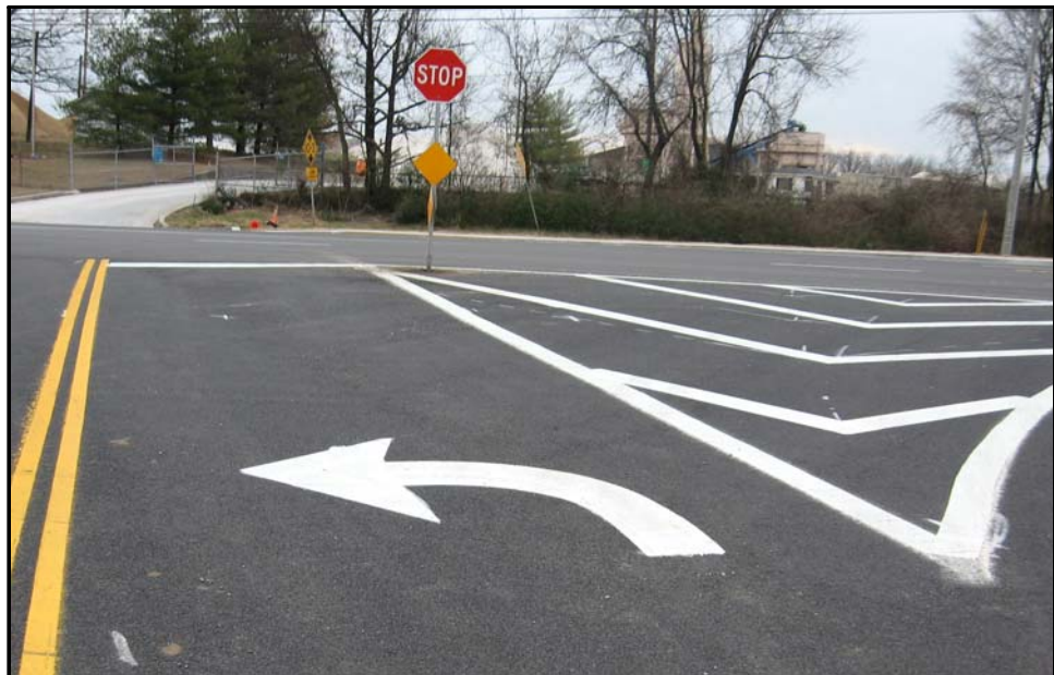
Special markings like this left arrow use pre-cut pieces for ease of installation.
