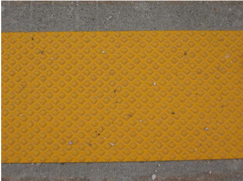
This yellow 6-inch wet reflective tape features raised squares designed to provide increased retroreflectivity in wet conditions. This marking material is commonly used on PCC surfaces such as freeway ramps and bridge decks.
