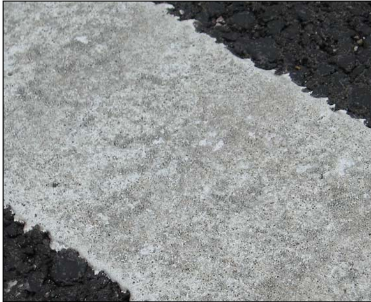
The small black dots visible on this white 6-inch sprayed thermoplastic marking are individual glass beads imbedded in its surface.
