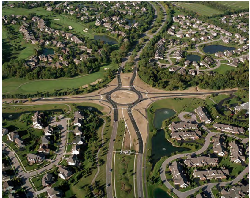
This multilane roundabout in Dublin, OH, was installed to address safety concerns at this location. (Photo credit: City of Dublin, OH)
