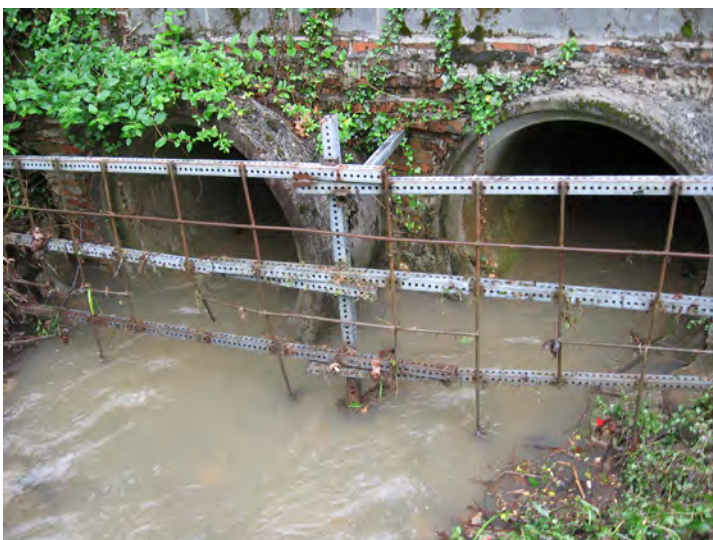
A cleaned drainage grate allows the maximum drainage flow to occur.
