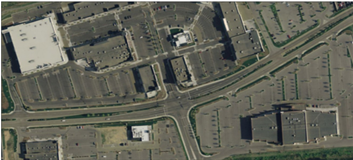
The Turkey Creek development in Knoxville and Farragut utilizes many access management techniques, including well-spaced signalized intersections and median crossings, right in / right out control for minor driveways, and sufficient corner clearance (source: maps.bing.com)
