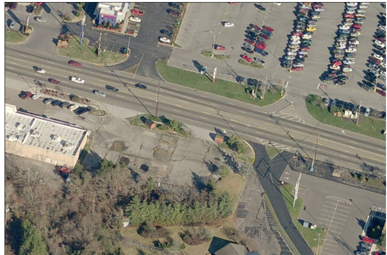
Driveway turn restrictions, such as these on Chapman Highway in Knoxville, limit potential conflicts near signalized intersections (source: maps.bing.com)
