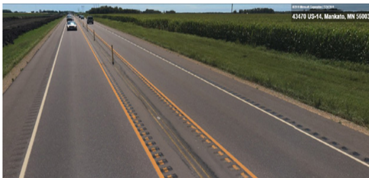
Use of Center Line Rumble Strips and Delineators to create a buffer on Highway 14 in Minnesota
