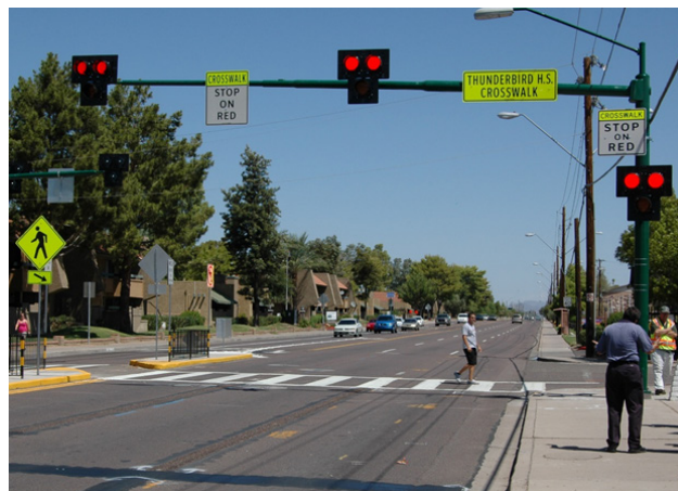
Pedestrian hybrid beacons (PHBs, also known as HAWK signals) stop vehicular traffic when pedestrians are present. PHBs rest in a dark state when not in use. Credit: www.pedbikeimages.org / Mike Cynecki.
