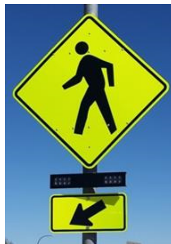
Rectangular rapid flashing beacons (RRFB) combine bright, rapidly-flashing lights with standard crosswalk warning signs and pavement markings to provide drivers with active warning of pedestrians crossing the street. Credit: Evaluation of Pedestrian Hybrid Beacons and Rapid Flashing Beacons, FHWA-HRT-16-040.
