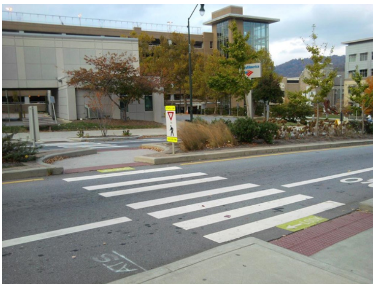
Pedestrian refuge islands reduce crossing distances and allow pedestrians to deal with only one direction of traffic at a time.
