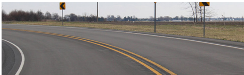
Signage, pavement markings and rumble strips are a few of the countermeasures listed on the Reducing Rural Roadway Departures initiative from EDC-5. (Source: FHWA)
